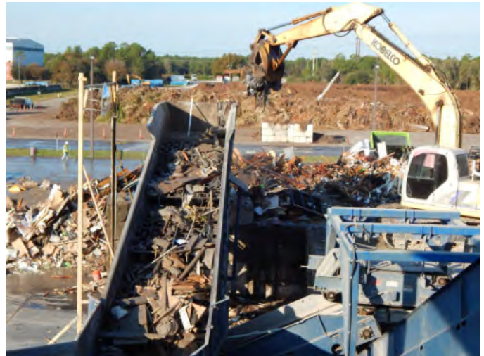
Figure 3.12 C&D Recycling Facility (Courtesy Lee County)
