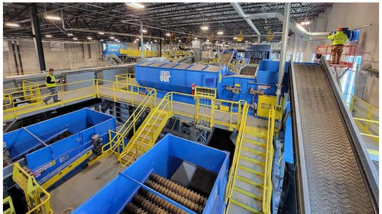
Figure 3.9 Typical MRF Facility (Courtesy CP)
