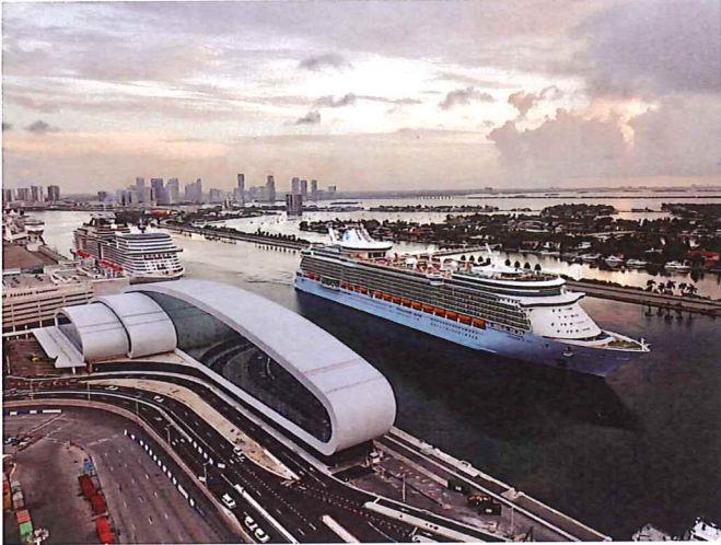
Figure 2: Photograph of Cruise Terminal B at PortMiami, which received LEED Gold certification in November 2021.
